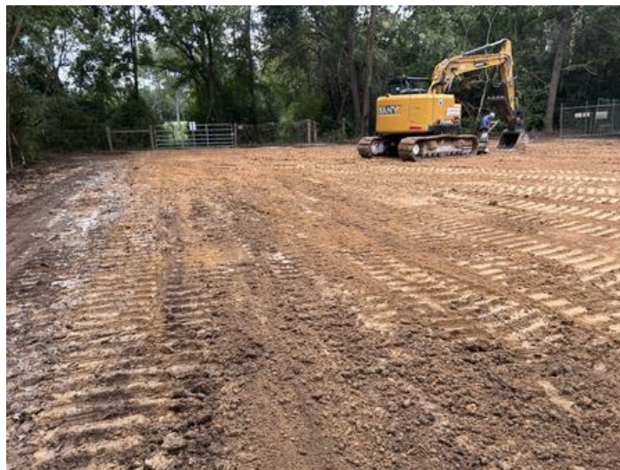
September 13, 2024 Water Plant Site Clearing
