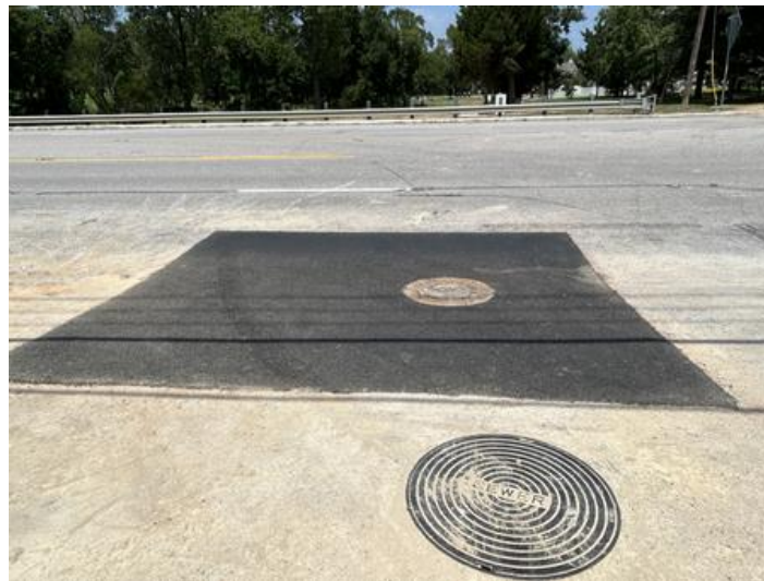
August 23, 2024 New Asphalt along SH 105
