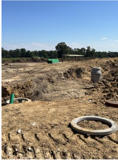
September 12, 2024 Cleared Site and Sanitary Sewer Installation
