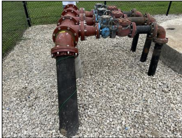
Lift Station Discharge Header Piping
