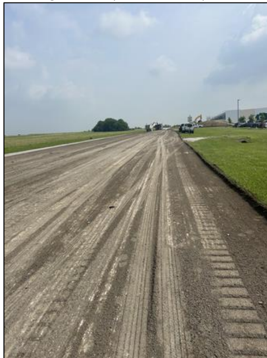
May 21, 2024 Existing Asphalt Removal
