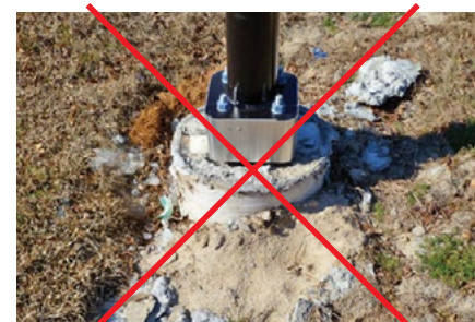
NOT Acceptable Footer Detail
