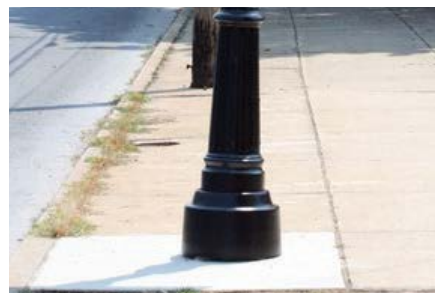
Acceptable Footer Detail
