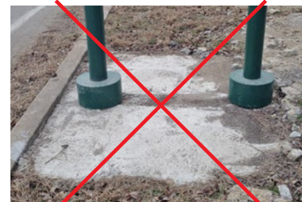
NOT Acceptable Footer Detail
